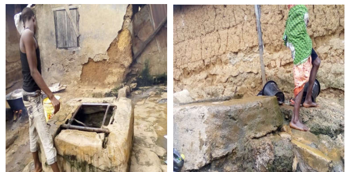
Plate 1 and 2. Unprotected Drinking Water Sources at Atikanakan area of Ado-Ekiti
