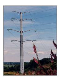
Ce pylône 2 x 220 kV Height: 40 meters Number of sections : 7 Load : 42 tonnes Calculated with a deflection limit of 4.5% ELU
