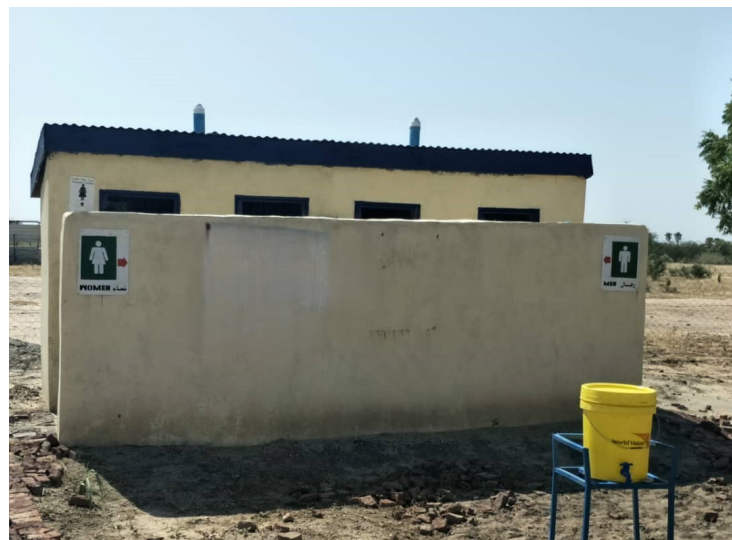
Plate 6. 1: Four stances sex segregated VIP latrine shared by both staff and patients with handwashing facility.
