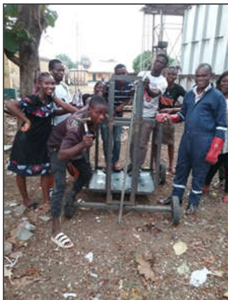
Figure 4b. Researcher and students in making of chassis for brick-built kiln (Ejiogu, 2021)
