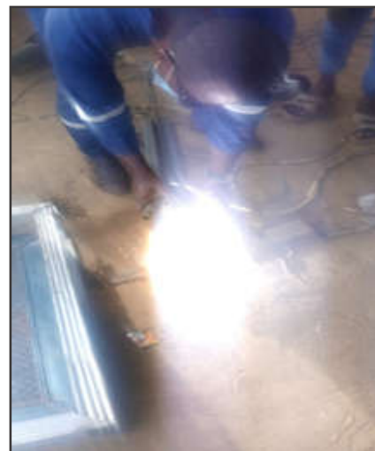
Figure 3a. Welding of iron parts together (Ejiogu, 2021)
